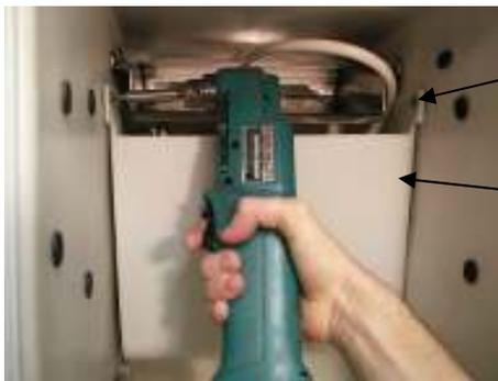
Remove the two screws and spacers at the reservoir
